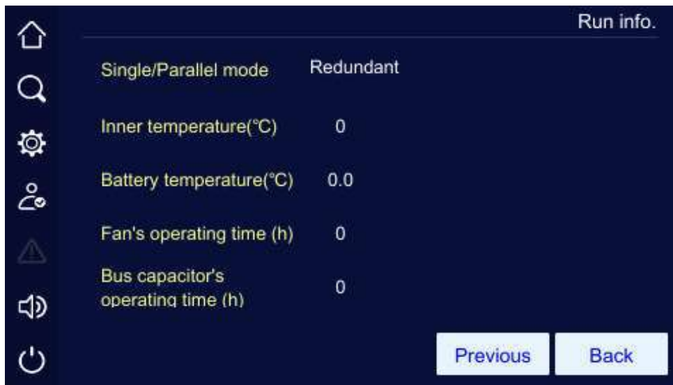
Working status page 2 (parallel UPS)
